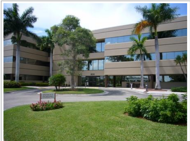
Commons V Medical Office Building, Naples, Fla.
